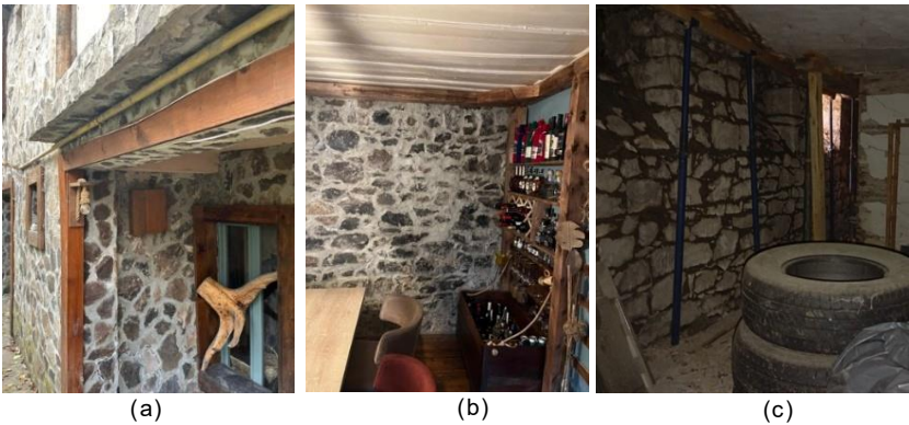
Figure 7. Stone cladding and wooden additions on the exterior façade for aesthetic purposes (a), wooden reinforcements and exposed load-bearing wall with removed plaster in the dining room interior (b), temporary reinforcements made in the basement (c). Source: Photograph by the first author (2024).
