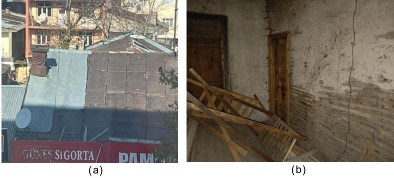
Figure 5. Roof covering constructed in accordance with the original design and decorative sheet-metal chimney cladding (a), and the interior wall on the ground floor constructed with the çakatura/bağdadi technique, with the plaster removed (b). Source: Photograph by the first author (2024).
