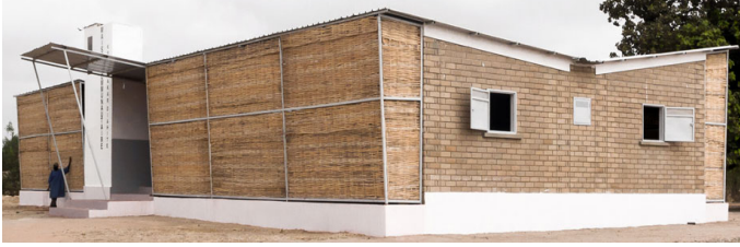
Figure 12. The H2OS project is a prototype house constructed of compressed earth block, that can harvest and store water supplies for all domestic uses and to integrate the scarce water resources in a few artificial walls ("Category: Compressed Earth Block", 2021).
