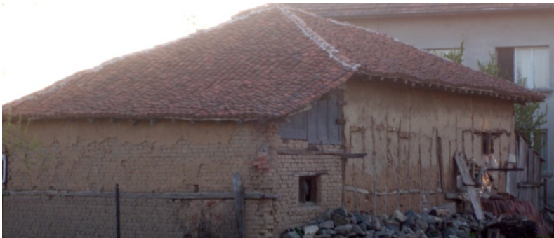
Figure 6. Masonry and wooden frame structural systems in an adobe building
