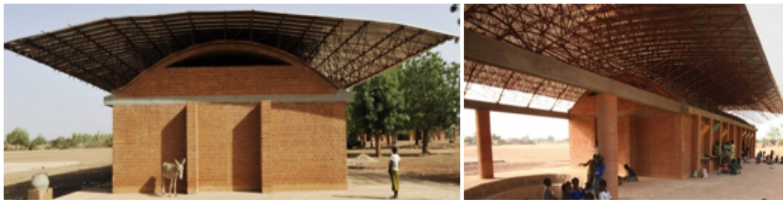
Figure 11. A modern building design in which steel space frame as a roof, reinforced concrete columns and compressed earth blocks are used together (Slessor, 2009)
