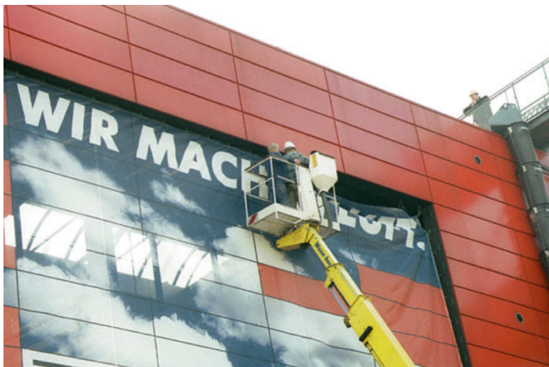
Figure 6. Facade cladding elements of infobox (Heiko Burkhardt, 2001)
