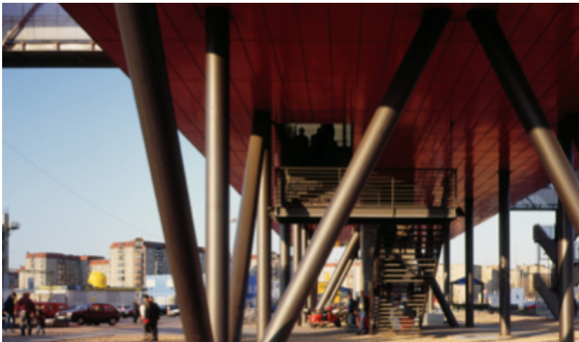
Figure 5. Infobox structural system elements in ground level (Schneider-Schumacher, 1995)
