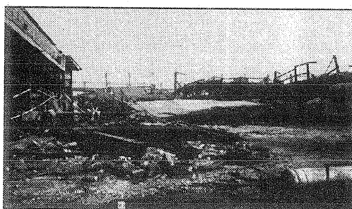
Figure 7. Damage occurred in The Railway Car Factory of TCDD with steel frame in Adapazari
