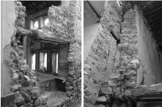
Figure 11. Building envelopes of Traditional Antakya Houses
