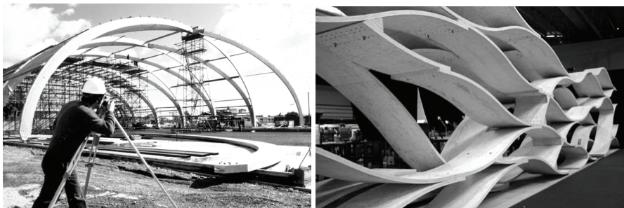
Figure 3. Curvilinear forms with glued laminated timber
