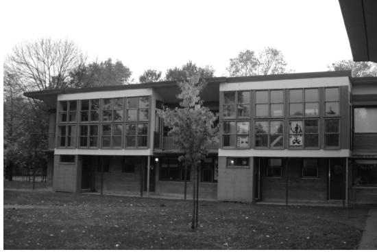
Passive solar gain is provided by windows with reused frames (Yilmaz).
