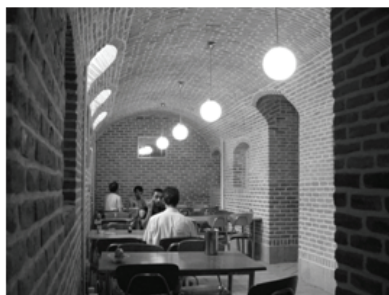
Figure 4. Thick walls provide a very good thermal protection
