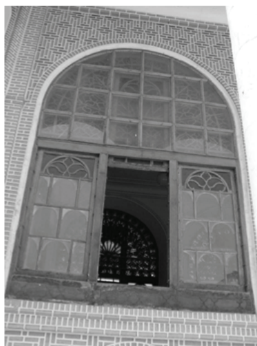
Figure 6. Colored glazing to moderate heat gain and loss by radiation
