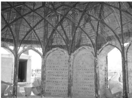
Picture 4. One type of light cassoon under construction.
