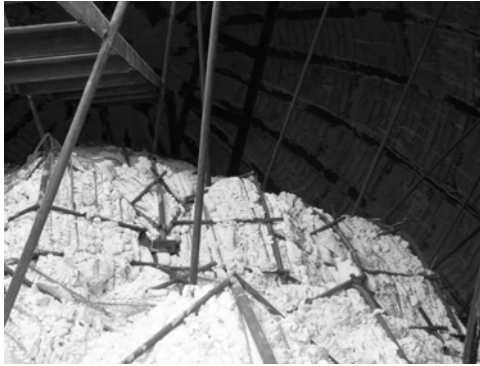
Picture 8. Back of one type of light cassoon (muqarnas) after construction.
