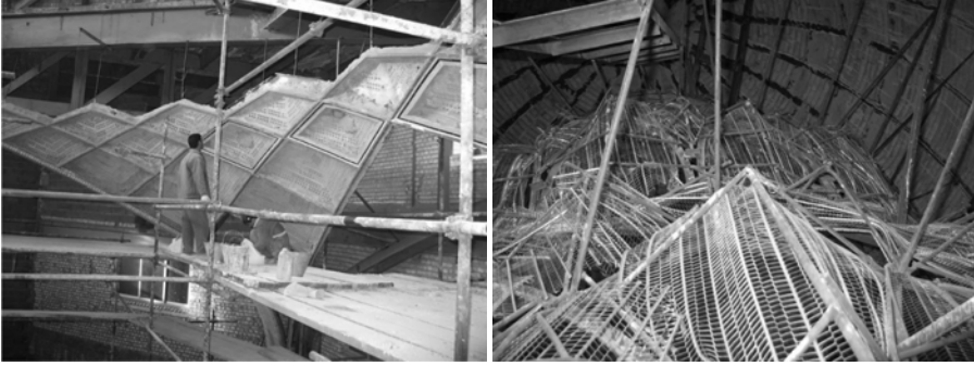
Picture 6, 7. Other type of light cassoon under construction; Back of one type of light cassoon (muqarnas) under construction.
