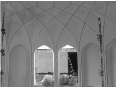
Picture 5. One type of light cassoon after construction.
