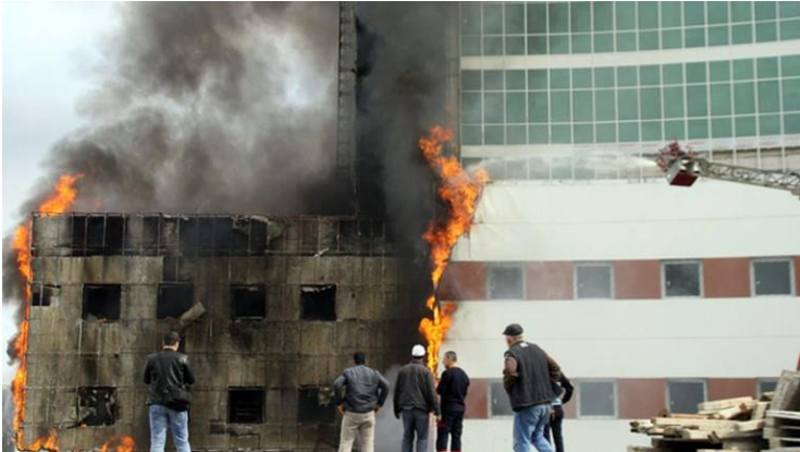
Figure 5. Fire Caused by Insulation Material
