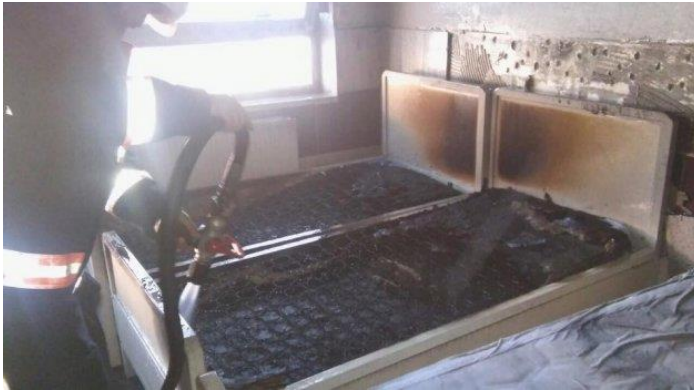
Figure 6. Post-Fire Condition of Patient Room without Fireproof Material
