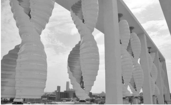
Figure 10. The Largest Building-Integrated Wind Power System in The U.S. is Now Spinning on the Roof of the Oklahoma Medical Research Foundation.
